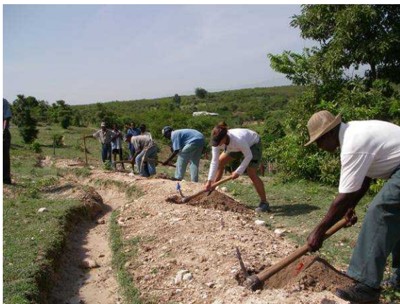
Figure 2. Volunteers digging a row of holes just below a contour canal.
