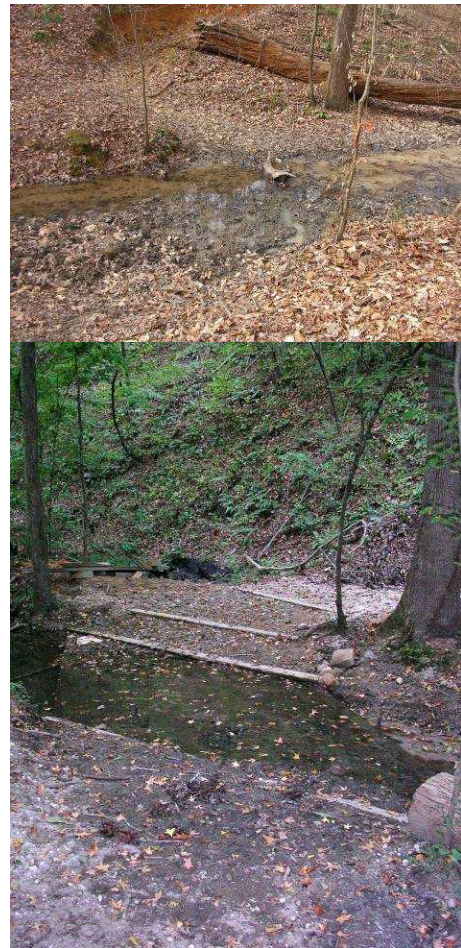
Figure 4. (Top) A poorly located stream crossing with no natural armoring on access or substrate leading to mucky conditions at the edge of the stream, (Bottom) Commonly used low water crossing design -- trail access to the stream has been hardened as well as the stream substrate.
